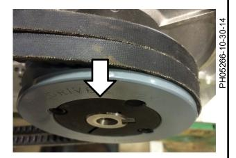
8. Install belts to the new generator and engine.
